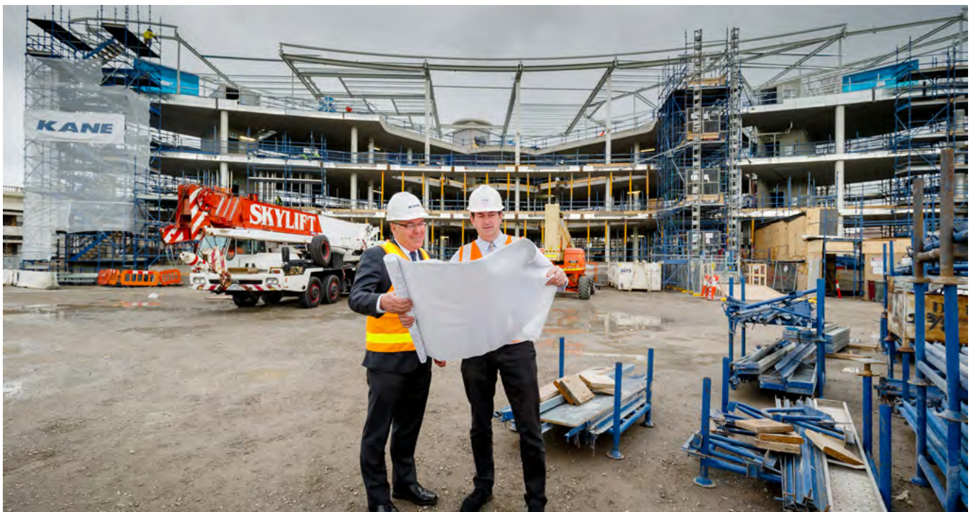
Mr Roy Kelley, Headmaster (left) and Mr John Phillips, Property Manager, inspect the Geoff Handbury Science and Technology Hub building site. The five levels (including the basement level and a partially enclosed roof level) are now in place. The next stages in the programme, once the roof is completed, are the installation of the steel façade framework, the external cladding and windows, then rough-in of the internal services with internal fit-out to follow that.
